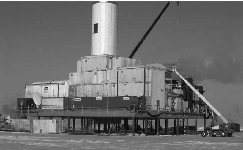
Arctic Drilling Platform at a site 60 miles west of Deadhorse, Alaska. Photo: Department of Energy Photo
