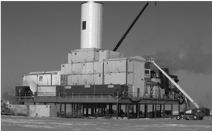
Arctic Drilling Platform at a site 60 miles west of Deadhorse, Alaska. Photo: Department of Energy Photo
